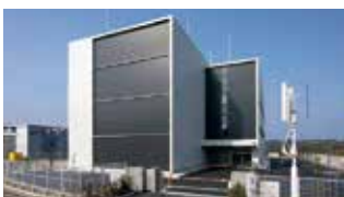
● Okayama Data Center
