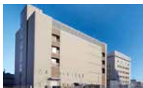
● Shizuoka Data Center
